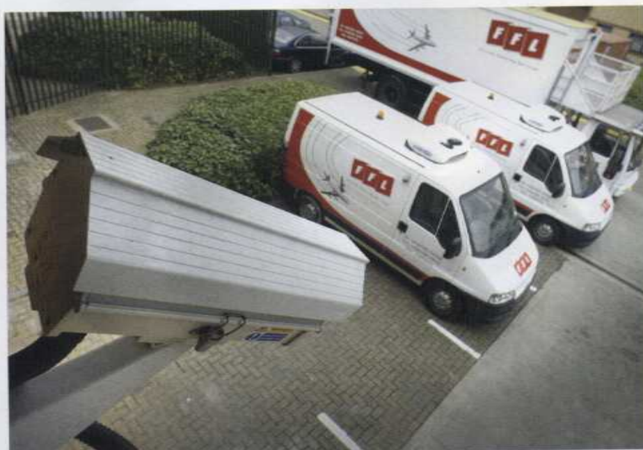
Cameras monitoring the lorry parking area are permanently set at a rate of six fps.
